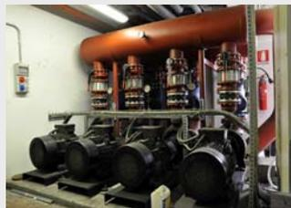
Ex Istituto Sieroterapico Milanese – Water to air heat pumps EQV series operating for the internal premises and detail of the pumping station.
